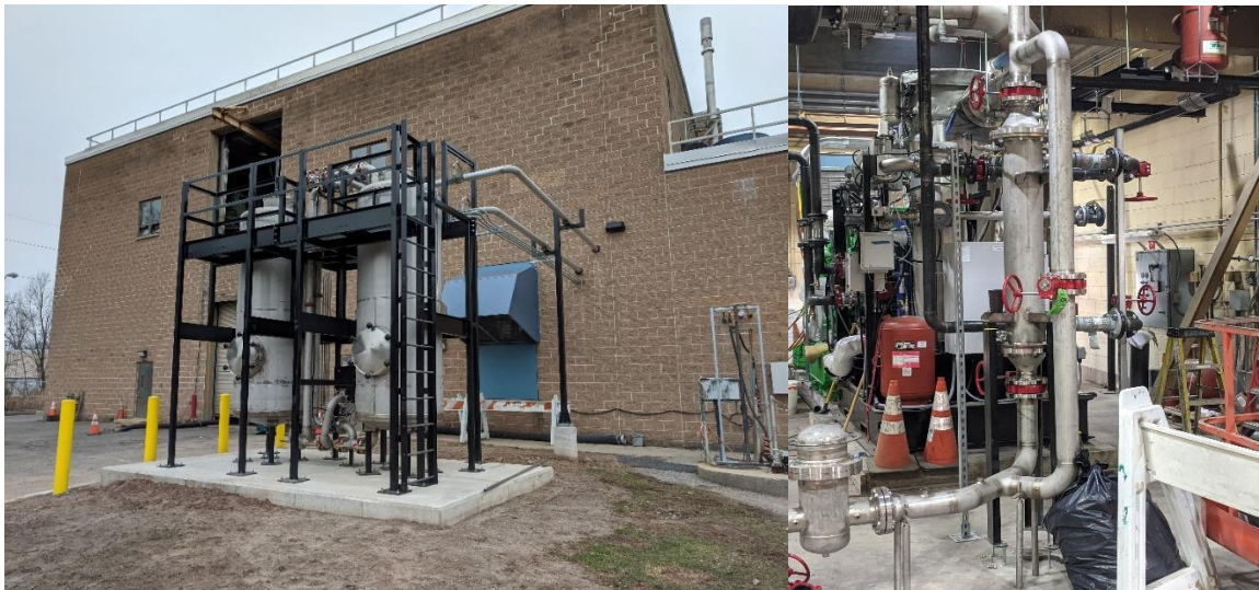
Figure 5 Siloxane Filter & Gas Preheat HX
