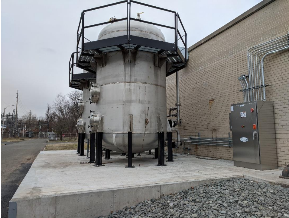
Figure 3 Drying Skid
